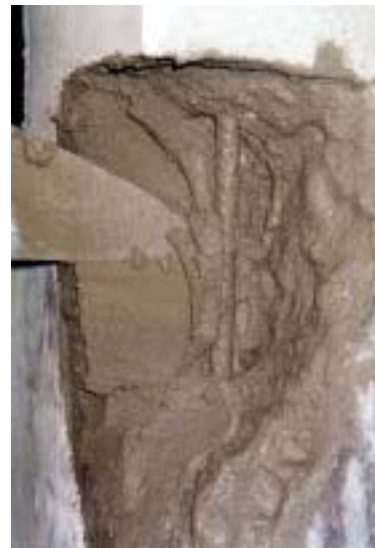
Apply the mortar
