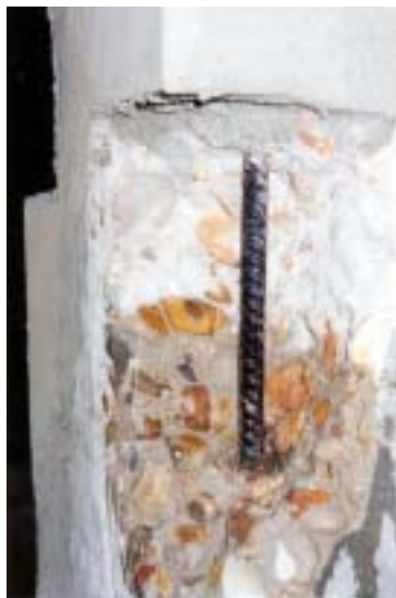
Damp the surface
